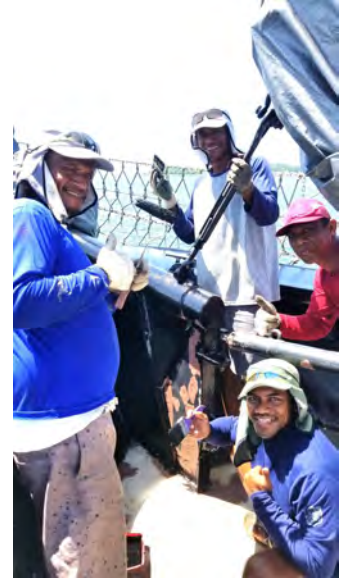
The crewmen painting the forecastle bulwarks and bowsprit after all the welding was finished.
